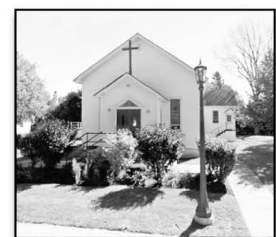
St. Andrews Church Sackets Harbor
